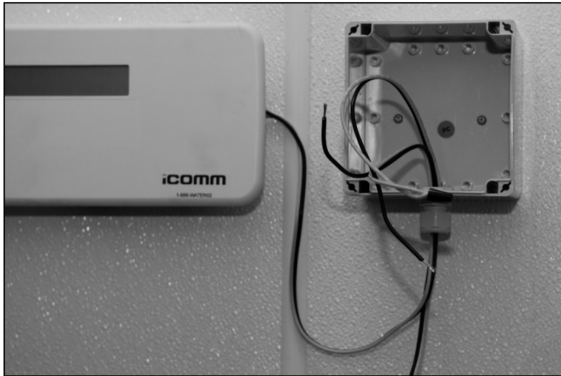
Alarm Box mounted - wiring routed inside enclosure
